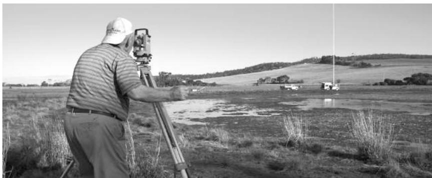
*Checking the mast at Sandford is vertical after replacing several sets of guy wires*
